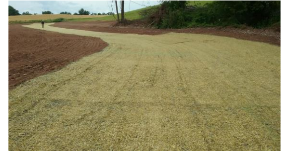
Newly constructed grass waterway
