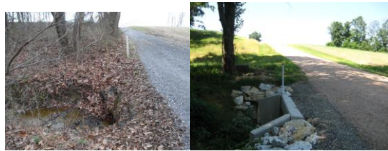
Culvert crossing replaced on Bittle Road, Germany Twp from a 30 inch pipe to 9 foot wide box culvert
