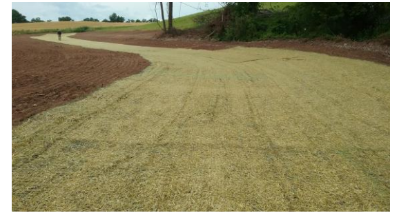
Newly constructed grass waterway
