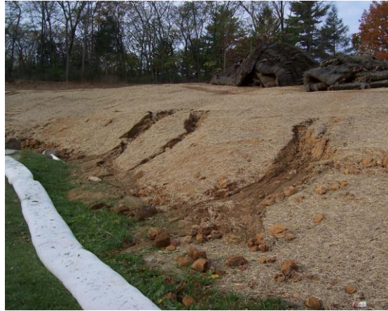
Active erosion is controlled with silt sock
